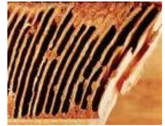
Termite Damage
